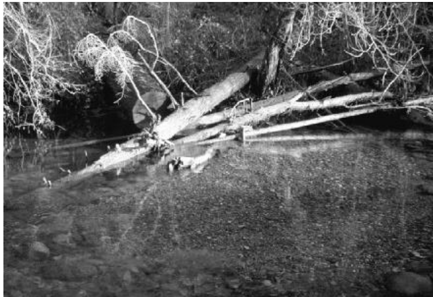
Figure A5-55. Complex log-cover structure in side channel of Elk Creek installed by Klamath National Forest. Photo courtesy of Al Olson. Circa 1991. Note spawning gravels adjacent to structure.
