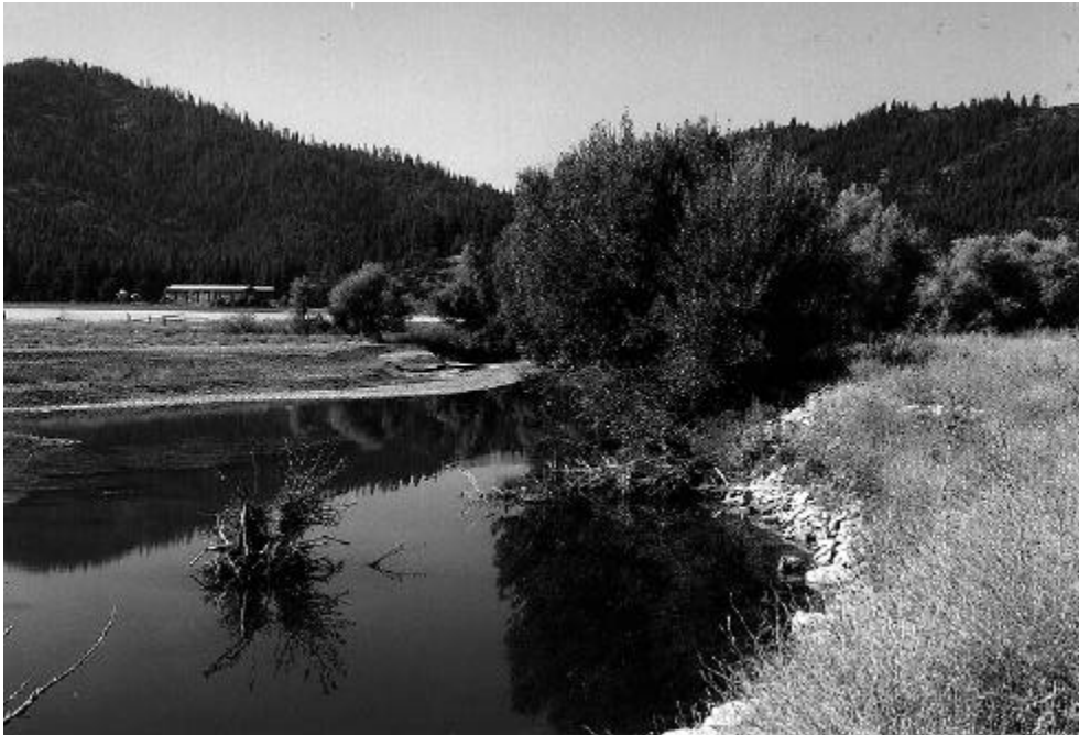
Figure A5-34. Bank stabilization project on the mainstem Scott River at Pastures of Heaven, combining rip-rap with tree planting. Photo July 1997.
