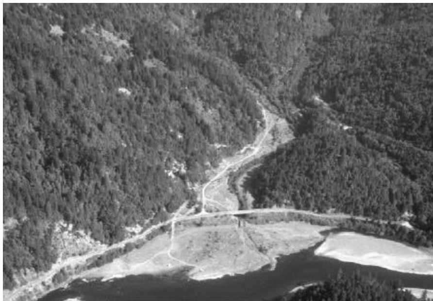
Figure A5-6. Cappell Creek represents a typical Lower Klamath Basin tributary delta. These large sediment deposits cause the streams to go under ground in late summer.
