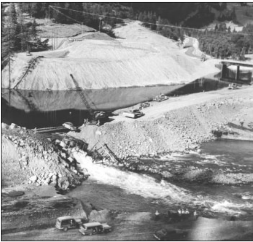
Cofferdam impoundment near Trinity Dam marking the beginning of flow regulation in 1958. Trinity and Lewiston dams were completed in 1964.
