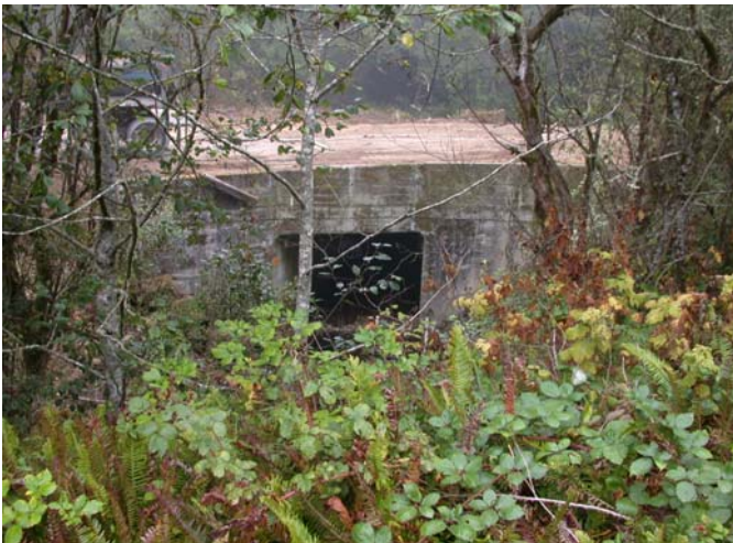
Pre-project view of box culvert looking upstream.
