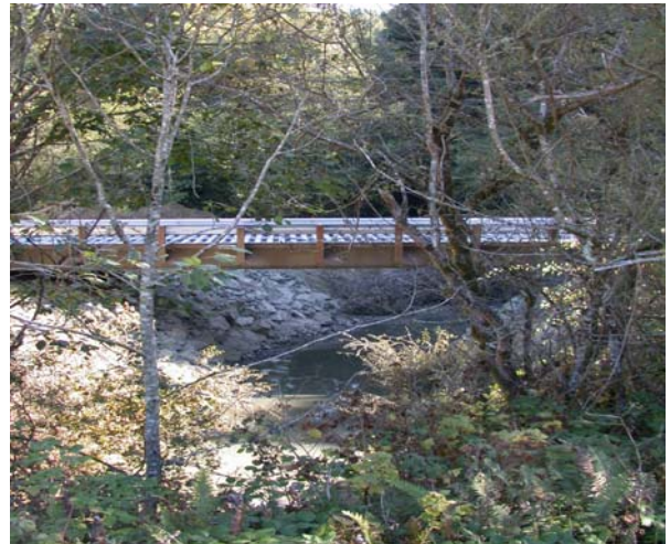
Post-project view of new bridge from same photopoint.
