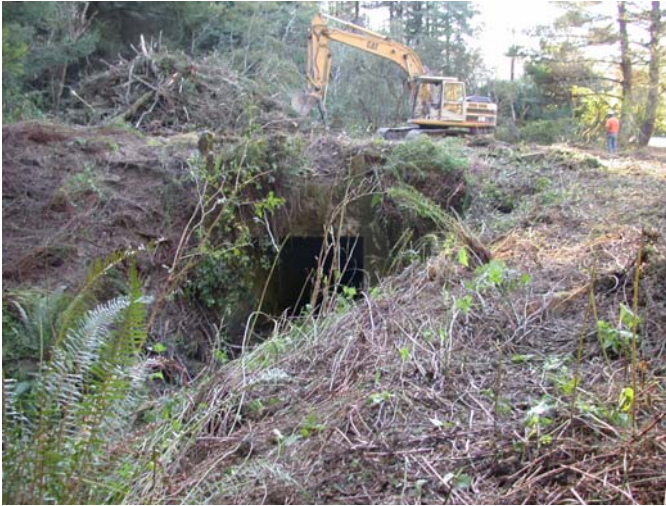
View of box culvert looking downstream while excavating the asphalt above.
