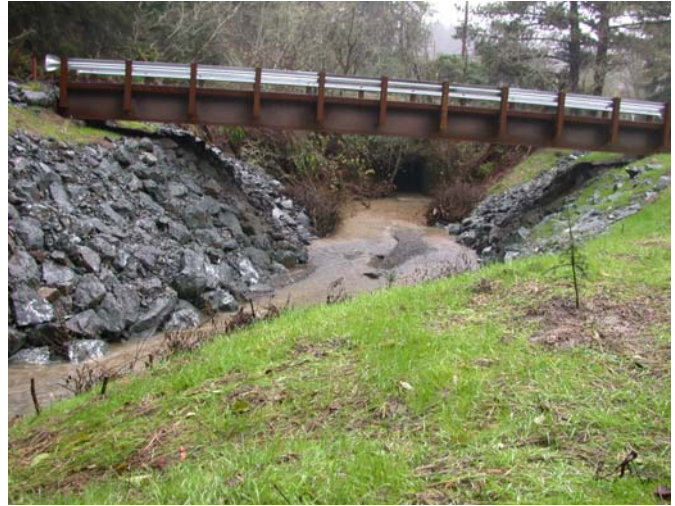
View of project site with culvert removed and bridge installed.
