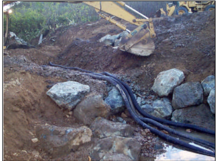
Installation of Vortex Weir
