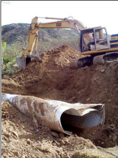
Culvert Removal
