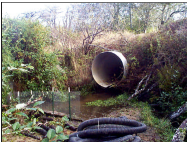
Failed Culvert and Fish Impediment
