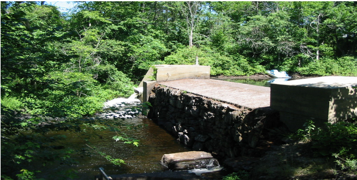
Coopers Mills Dam; July 2003
